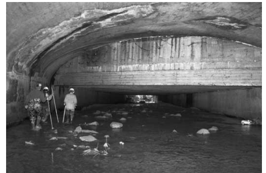
Our planning experts donned wading boots to investigate culverts that provide clues about the feasibility of "day-lighting" the Saw Mill River. Sections of the important waterway were paved over more than a century ago.
