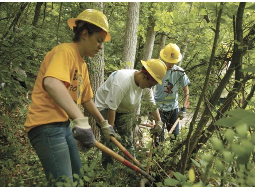
Members of the Beacon Environmental Stabilization Team (BEST) worked on preparing new trails at Madam Brett Park in Beacon, Dutchess County.
