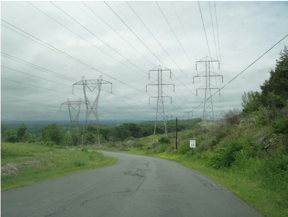
Shared ROW Town of Milan, Becker Hill Road
