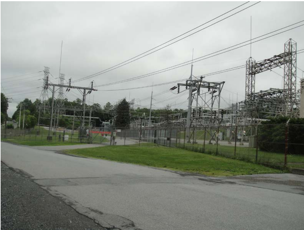
Pleasant Valley Substation
