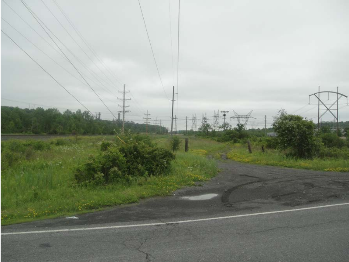
Leeds substation area
