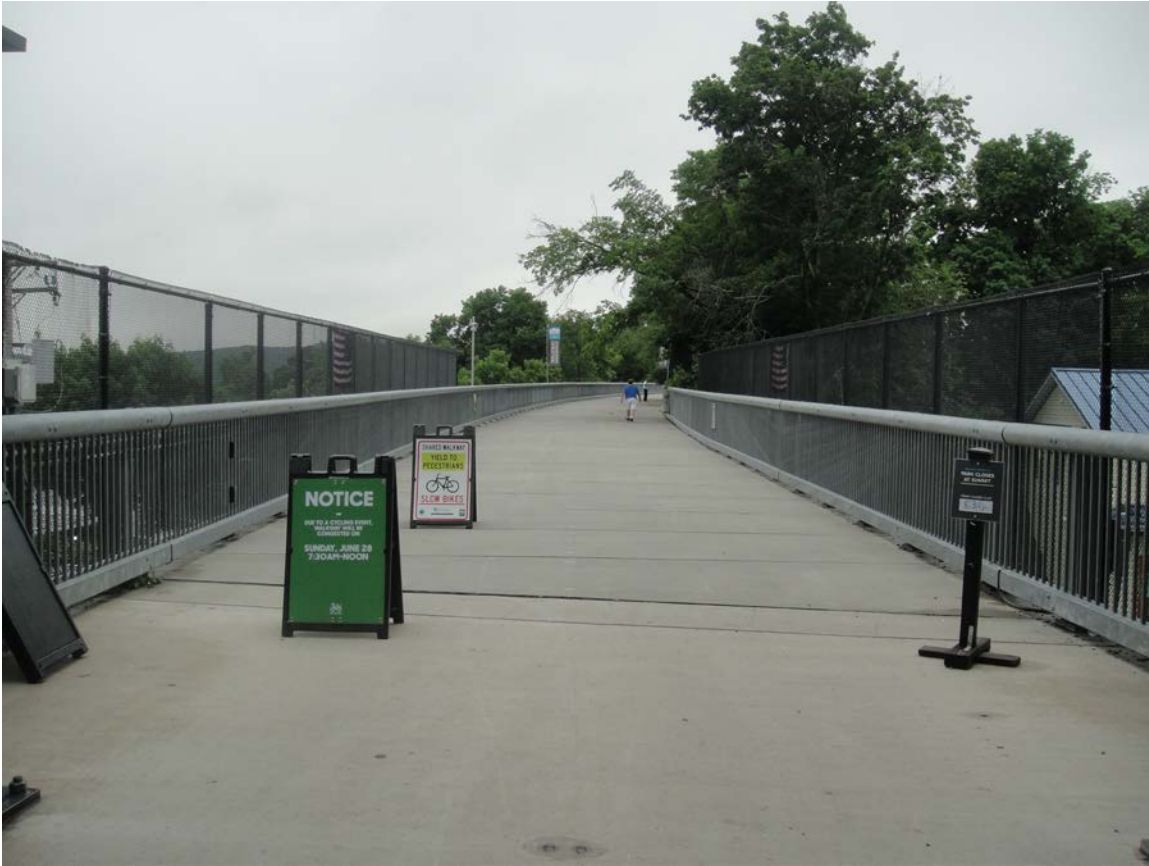
East side of Walkway over the Hudson, looking west
