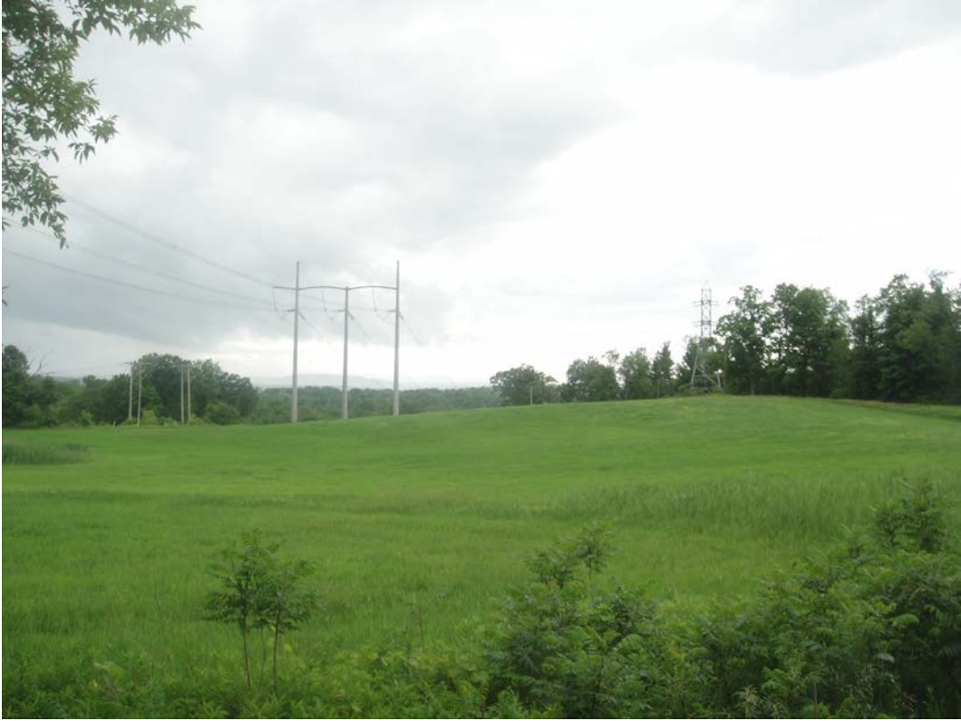
Knickerbocker/Muitzekill Road – Knockerbocker substation area
