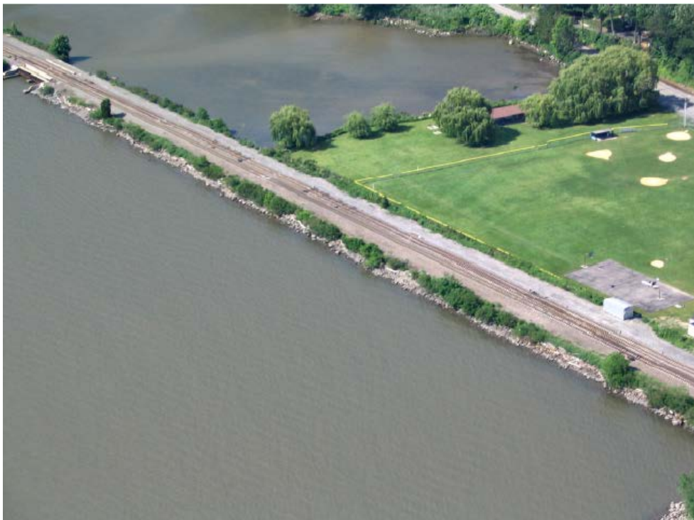
Figure 41: ESI 6B Riprap Shore on Hudson River
