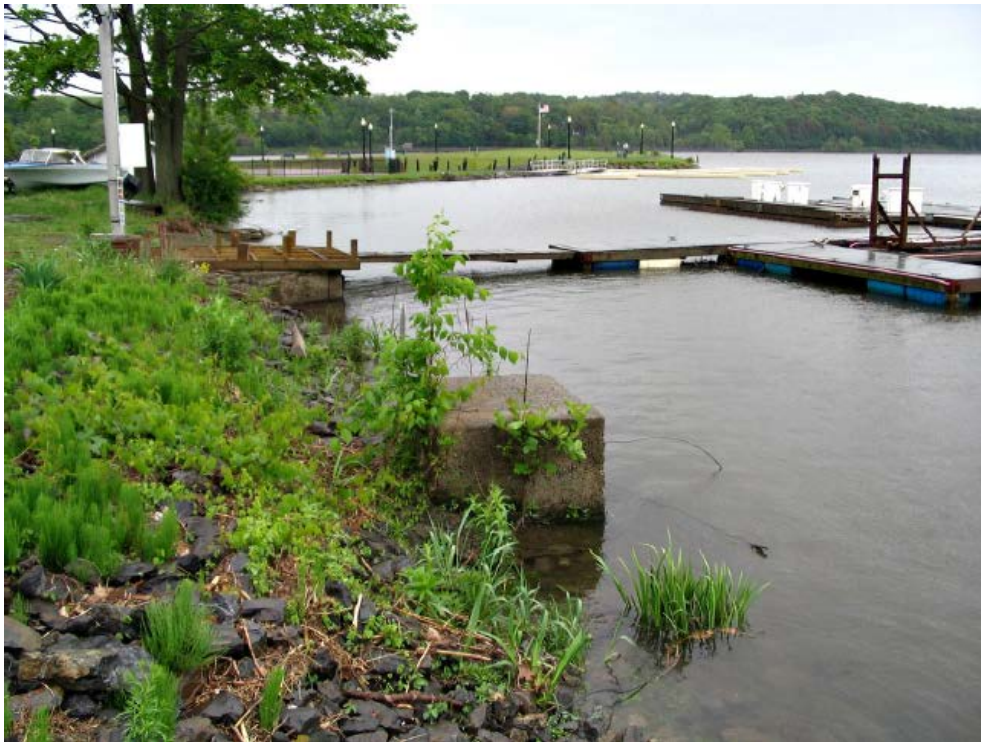
Figure 45: ESI 8C Sheltered Riprap on Hudson River
