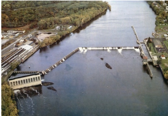
Figure 21: Troy Federal Lock and Dam 22
