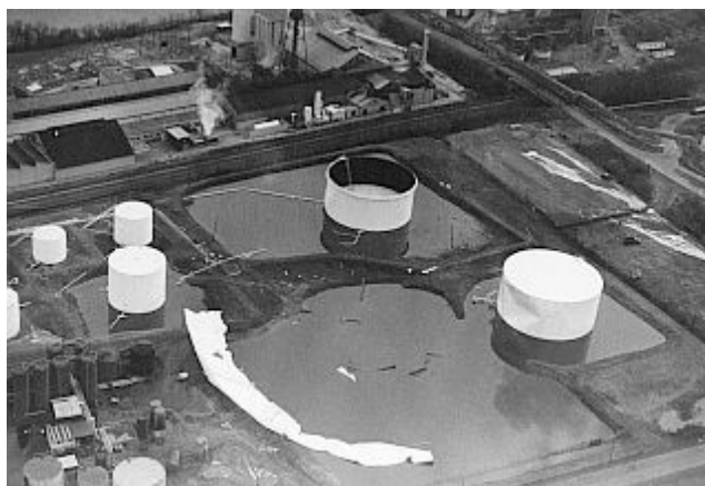
Figure 32: Aerial Photo of Collapsed Ashland Oil Tank
