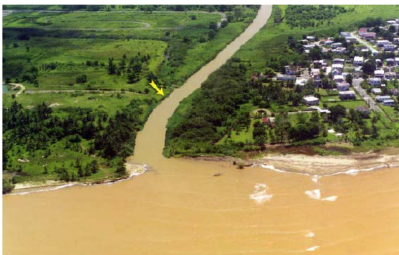
Figure 61: Sheltered, Vegetated Low Banks
