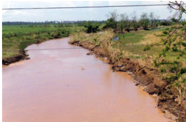
Figure 50: Exposed Scarps and Steep Slopes in Clay
