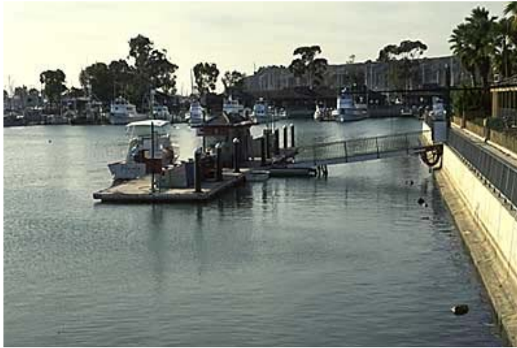
Figure 59: Sheltered, Solid Man-Made Structures
