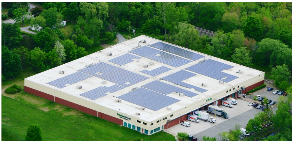
Central Valley, 531 kW
