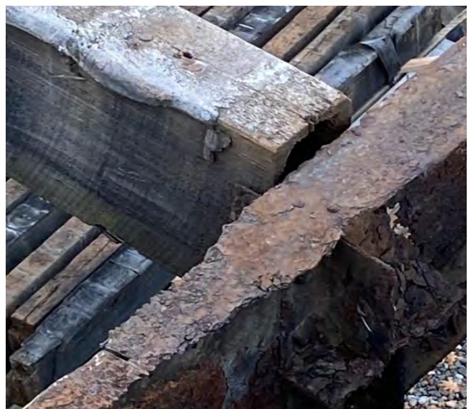
View of deteriorated steel floor beam and wood stringer prior to replacement
