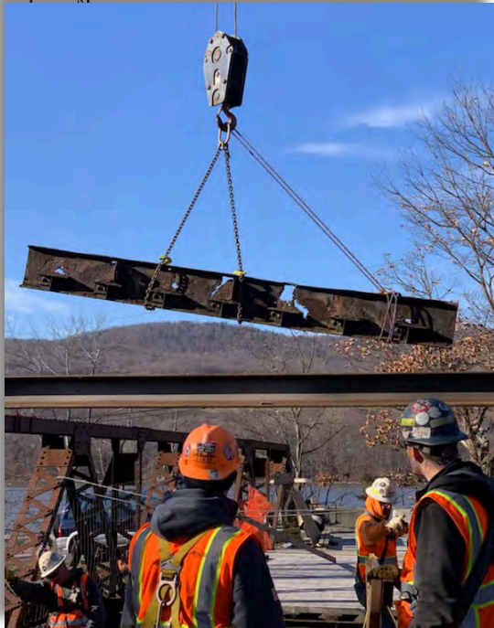
One of two seriously deteriorated floor beams being removed.
