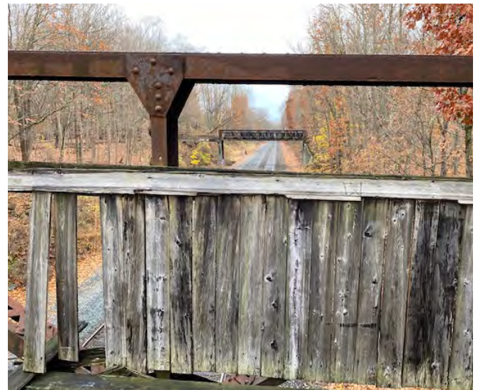
Deteriorating wood horse barrier - South Bridge in background
