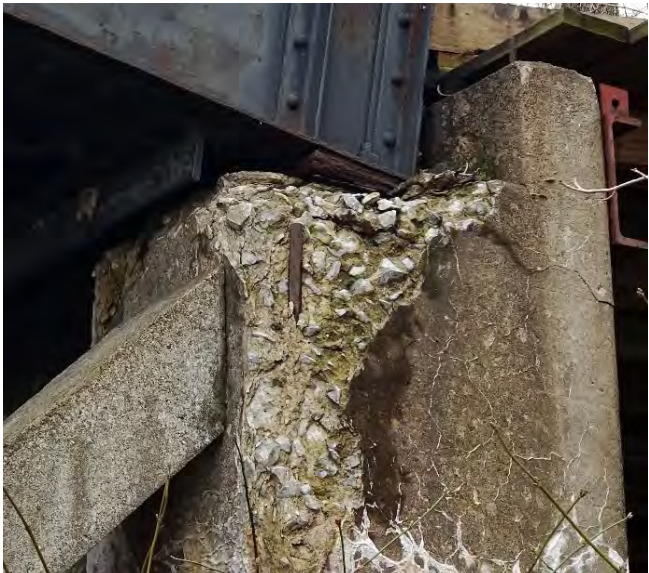
Eastern pier bearing with exposed rebar
