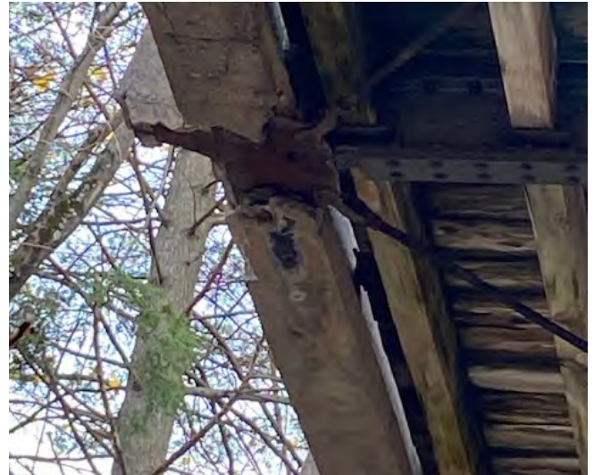
Failure of concrete cover at tie rod connection plate
