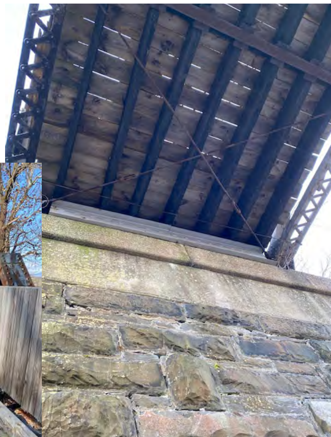
View of east abutment / truss interface
