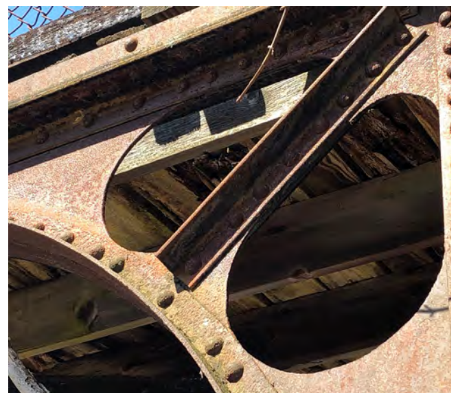
Truss / steel column transition
