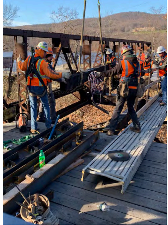
Harrison & Burrowes crew carefully removing wood stringers from the steel floor beams for reuse.
