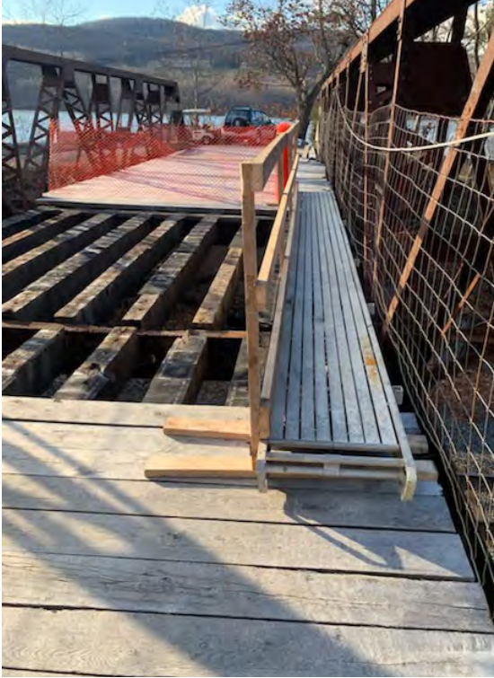
3 inch wood planks removed over Amtrak tracks revealing wood stringers and steel floorbeams
