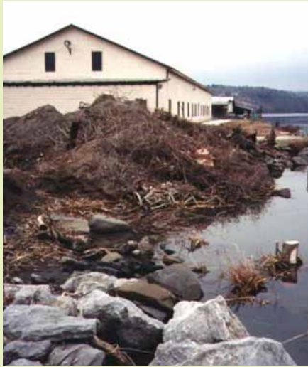
Shoreline before restoration.
