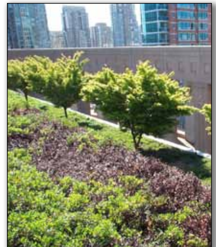
A rain garden as part of a vegetated swale effectively manages stormwater.
