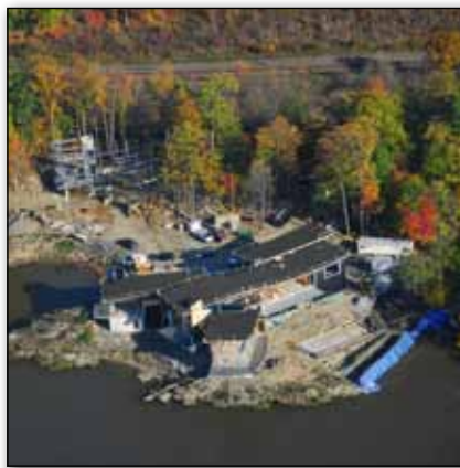
This home on the Hudson River with little setback and no vegetative screening mars visual quality.
