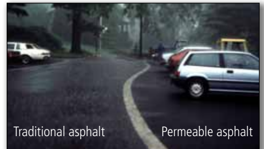
Permeable asphalt treatment of parking stalls.
