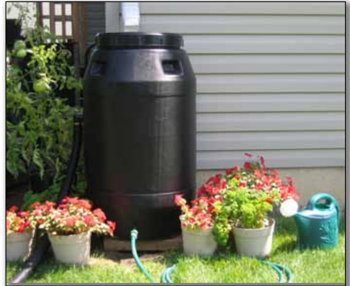
Rain barrels or cisterns capture roof run-off that can be used to water lawns and gardens.
