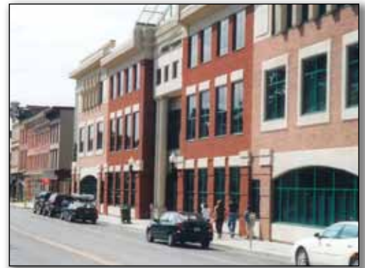
New buildings, such as these along Poughkeepsie's Main Street, reflect local scale and character.
