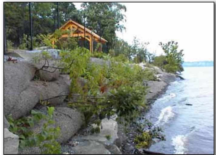
Installed vegetated shoreline stabilization treatment with native plant species, biodegradable soil bags, and a sloped shoreline.
