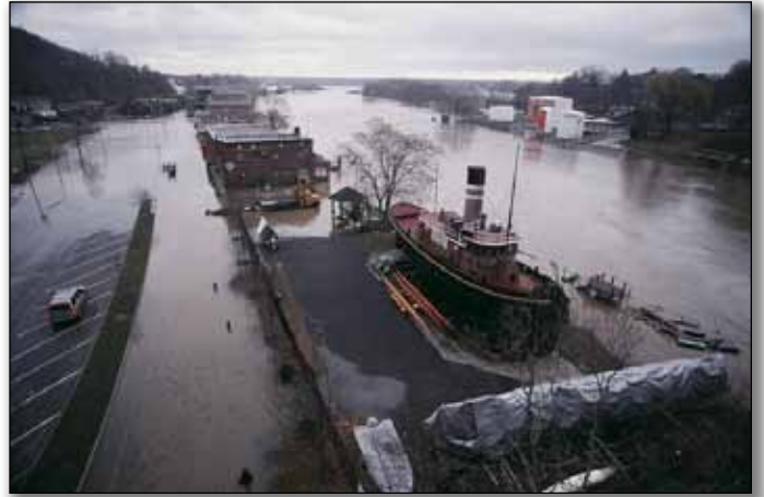
April 2005 flooding in the City of Kingston.
