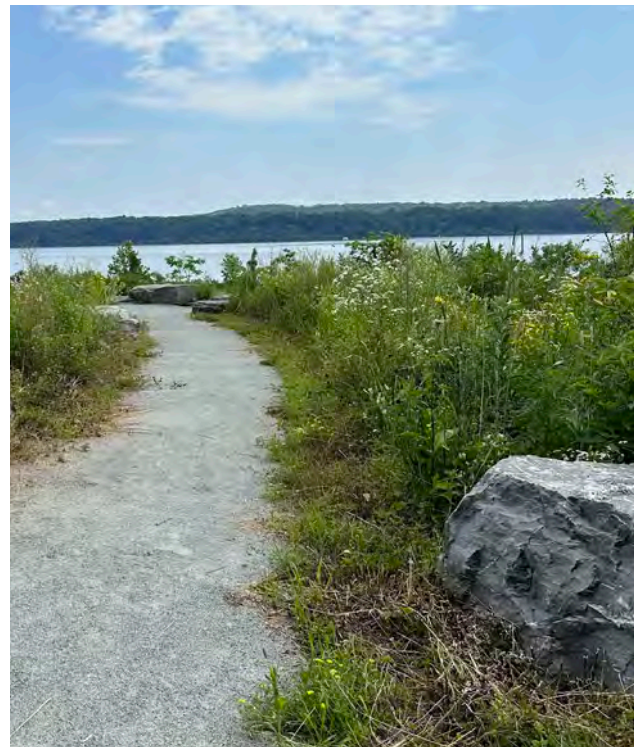
Figure 75. Example of compacted stone fines secondary trail with meadow planting and seating area, Sojourner Truth State Park. Source: OLIN.
