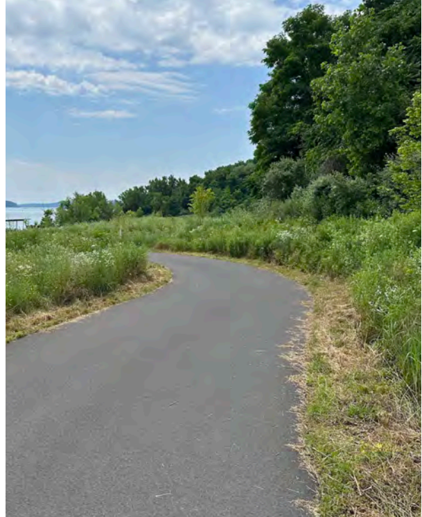
Figure 74. Example of 10' wide asphalt trail with nearby preservation area, meadow planting, and mown shoulder, Sojourner Truth State Park. Source: OLIN.
