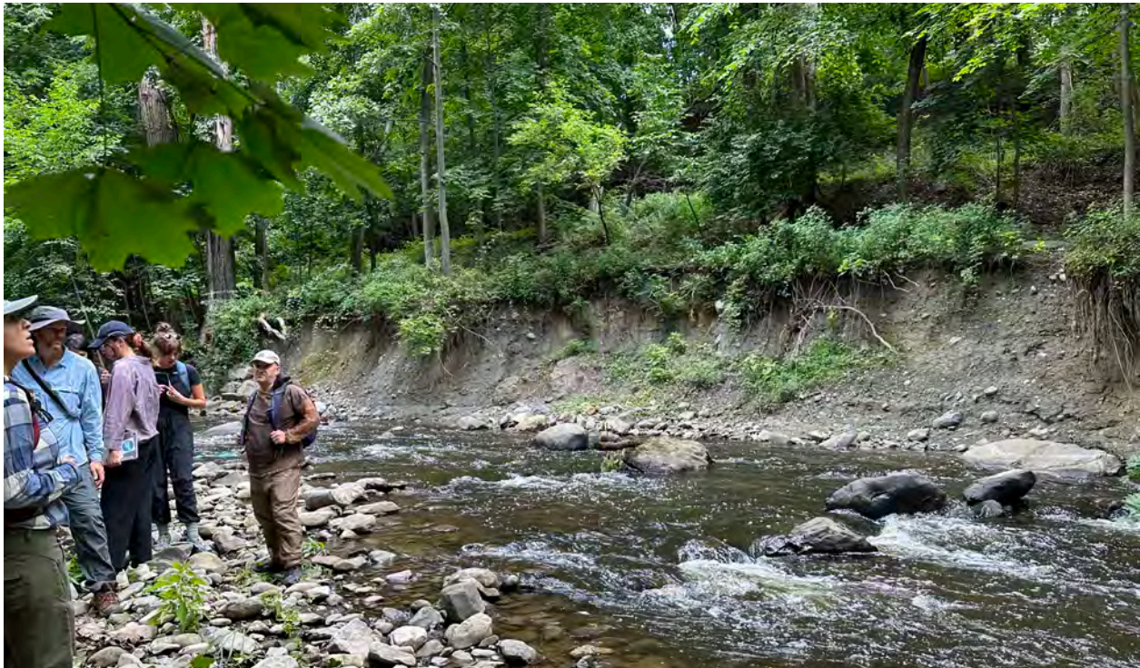
Figure 21. Eroded banks of the Quassaick Creek adjacent to an active industrial use. Source: OLIN.
