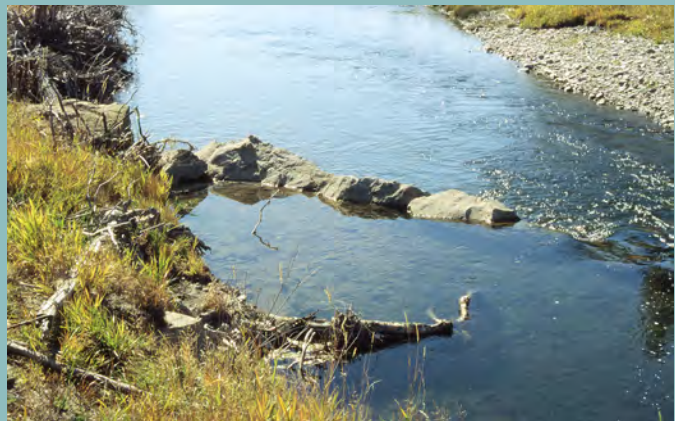
Figure 43. In-creek habitat enhancement - J-hook. Source: eDesign Dynamics.
