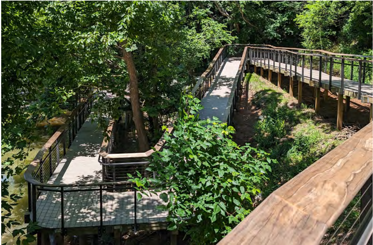
Figure 76. Elevated ADA-compliant accessible ramp; example of a potential access element with minimal forest disturbance proposed for the Mill Street Bridge Trailhead. Source: OLIN.
