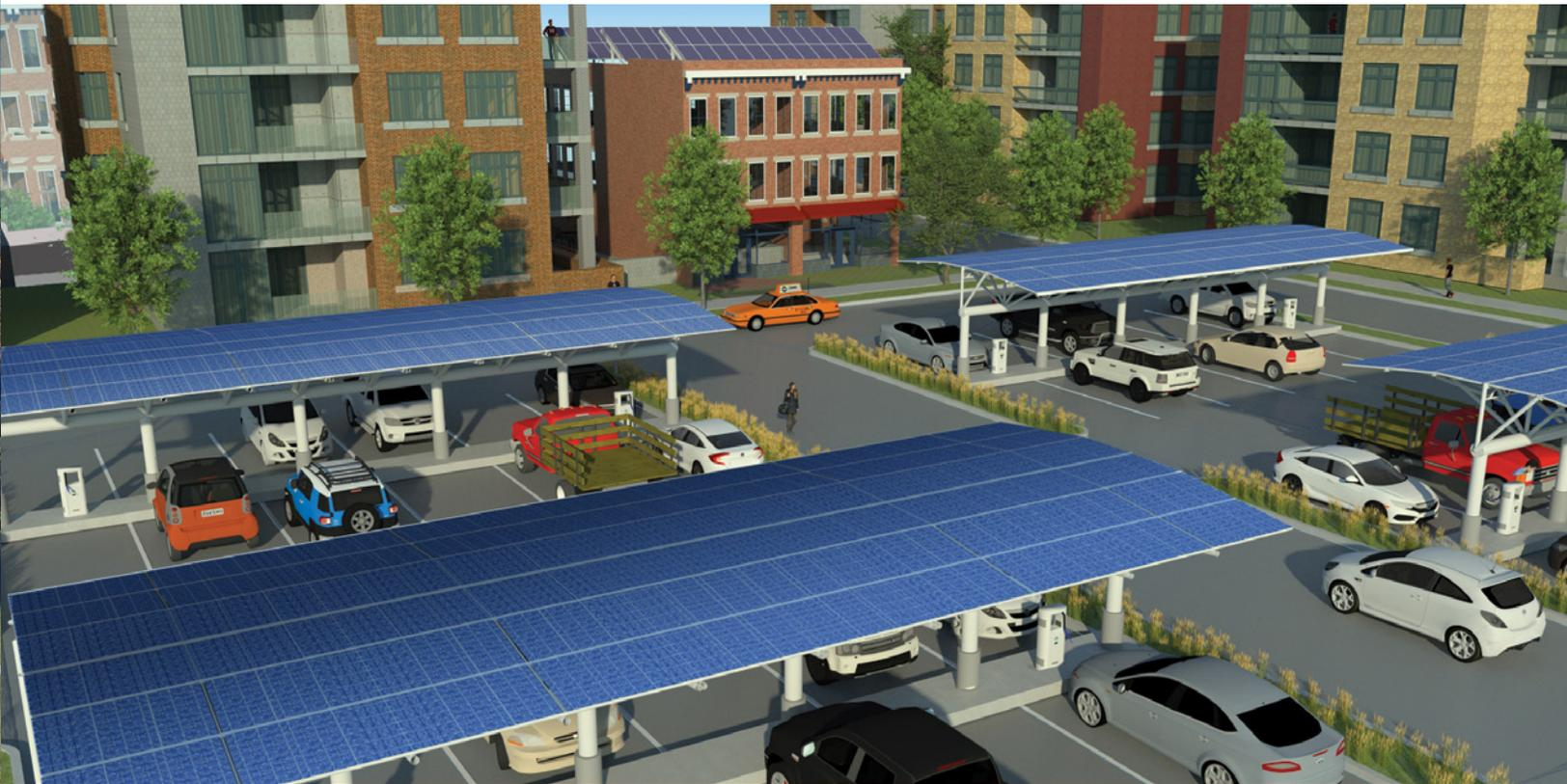
Parking lots and garages can offer ideal locations for solar installations because they often furnish the large, unshaded and unobstructed spaces optimal for such systems. Solar canopies in parking areas can provide shade and weather protection for cars parked beneath them as well as supply energy to electric vehicle-charging stations.
